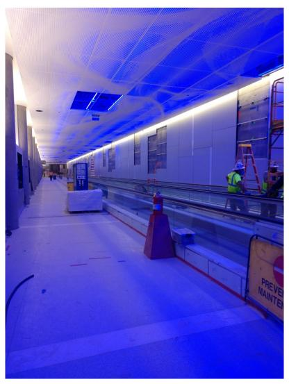
Pictured is a very long corridor, which is part of the Passenger Tunnel (PAX). To the right is a movable walk and to the left is a walkway for persons who want to walk the distance from Bradley West to the Midfield Concourse. On the wall to the right are panels where messaging and advertising will be located.
