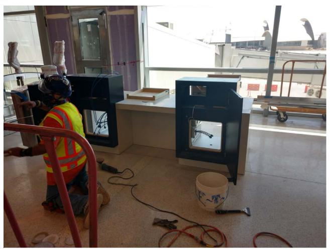
Pictured above is a workman kneeling at the left corner of the picture. Also shown is a check-in counter that is in the process of being installed. The picture shows a middle counter that can easily be approached by a wheelchair user and a higher counter on either side of the middle counter. A window and jet bridge are visible in the background.
