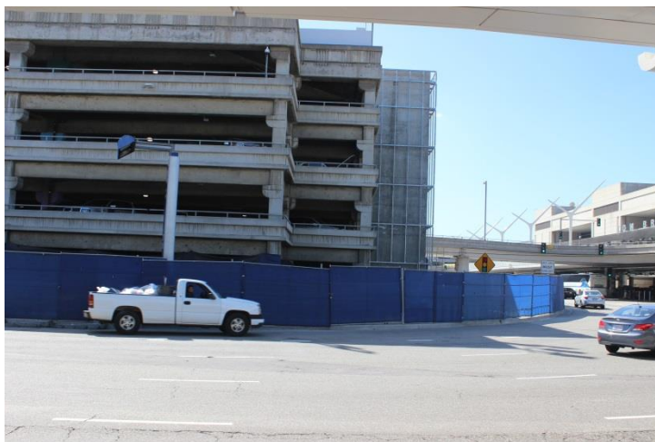
Metal panel installation has restricted the sidewalk and plaza at Parking Structure 3, while the left lane is occasionally closed.
