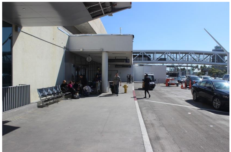
The construction barricades at Terminal 1 will be extended 120 feet in this direction in early April as renovation work shifts.
