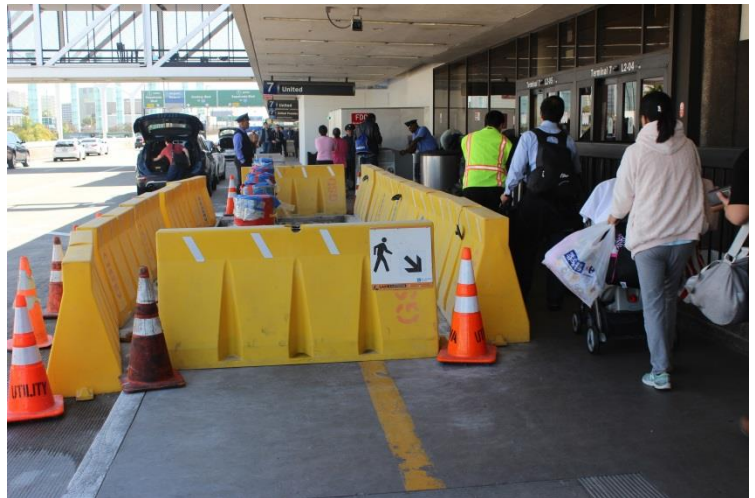
Security bollard installation is restricting sidewalks at several locations, including outside Terminal 7 (above).
