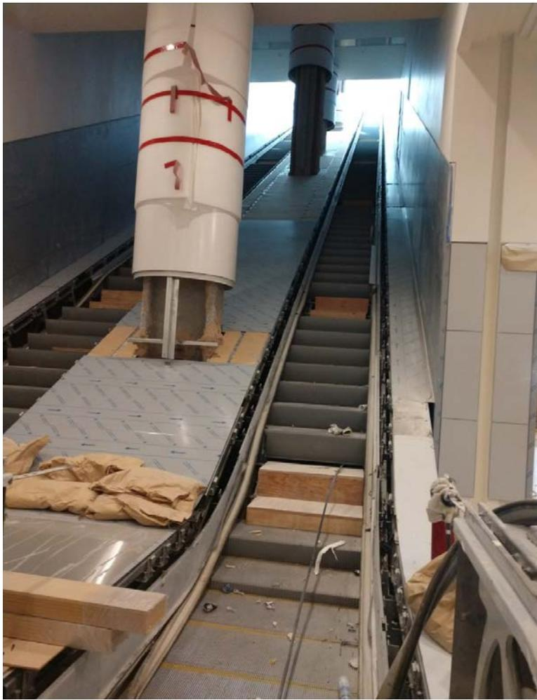
Pictured are two escalators and support beams in the center between the escalators. Escalators are under construction as are the beams and surrounding area is wrapped waiting for work to be done.
